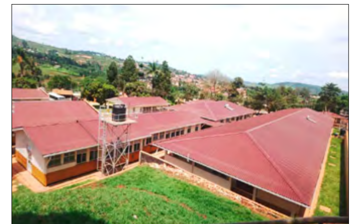
Overview of the hospital site showing various structures constructed
