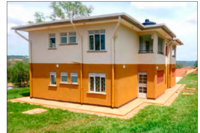
Housing facility with four apartments for medical staff at Kawolo
